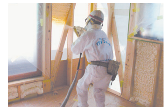
Spraying the AQUA FOAM insulation
