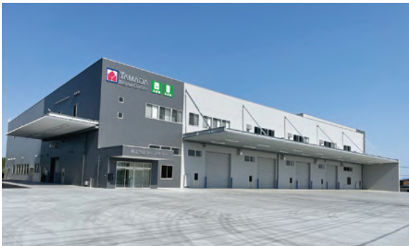
The new plant at the YAMADA East Japan Reuse Center Gunma Plant
