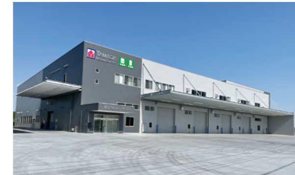
The new plant at the YAMADA East Japan Reuse Center Gunma Plant
