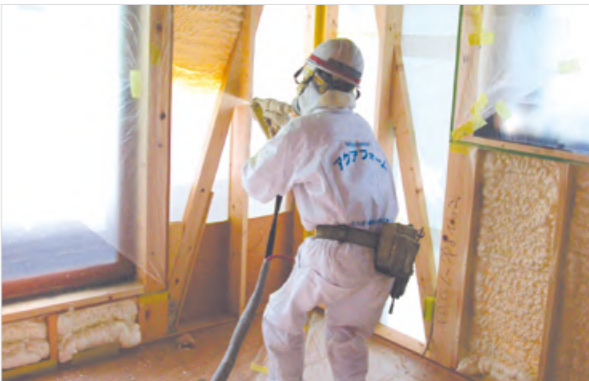
A worker sprays Aqua Foam into a wall
